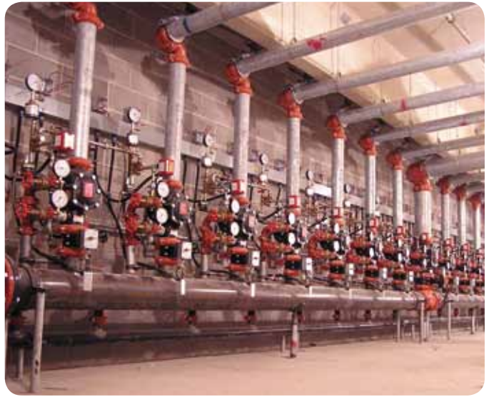
FireLock NXT Preaction System Check Valve† SERIES 769, PGS. 8-5-8-7
